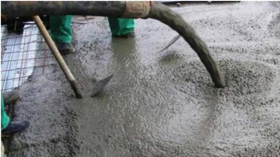
We established last month that water-cement ratios are key to understanding the potential quality of a concrete mix. However, we also discussed the lack of correlation between w/cm ratio and slump in today's concretes. How is that possible? Water reducers.
